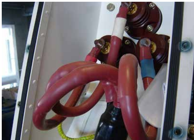
Figure 52 – Termination made without regard to dimensional instructions
