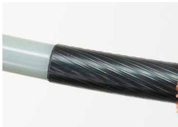
Figure 22 – Finished screen edge and smooth insulation surface
