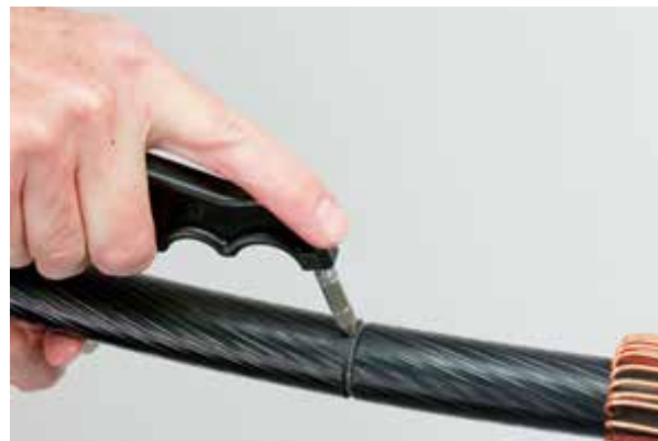
Figure 20 – Using a depth-guarded knife to score the screen
