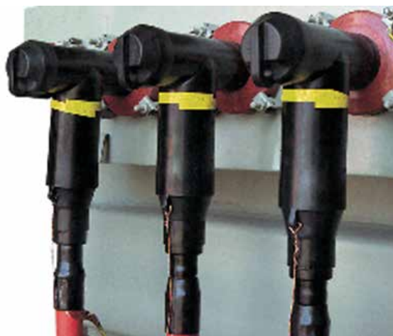
Figure 45 – Screened separable 'T' connectors (or 'elbows')
