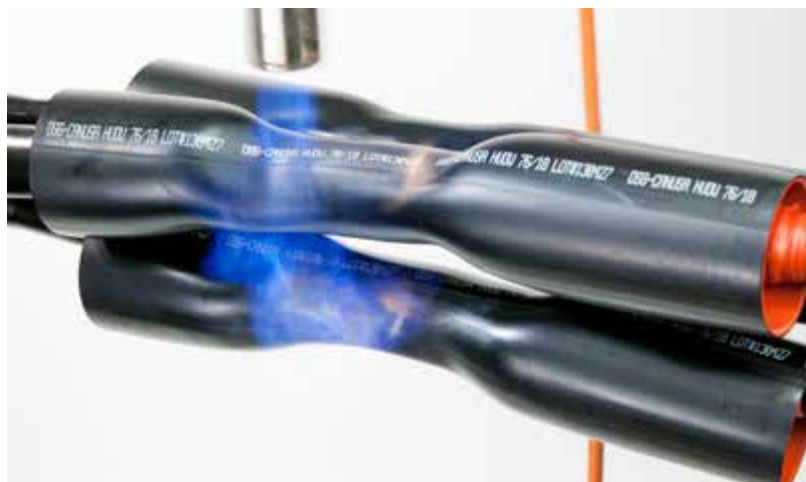
Figure 43 – Shrinking joint insulation/screening tubings
