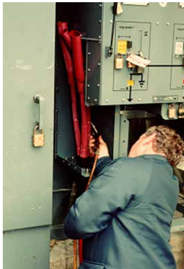
Figure 14 – Inadequate installation space between substation equipment
