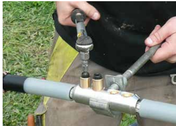
Figure 39 – Bolted connector with hexagonal socket screws
